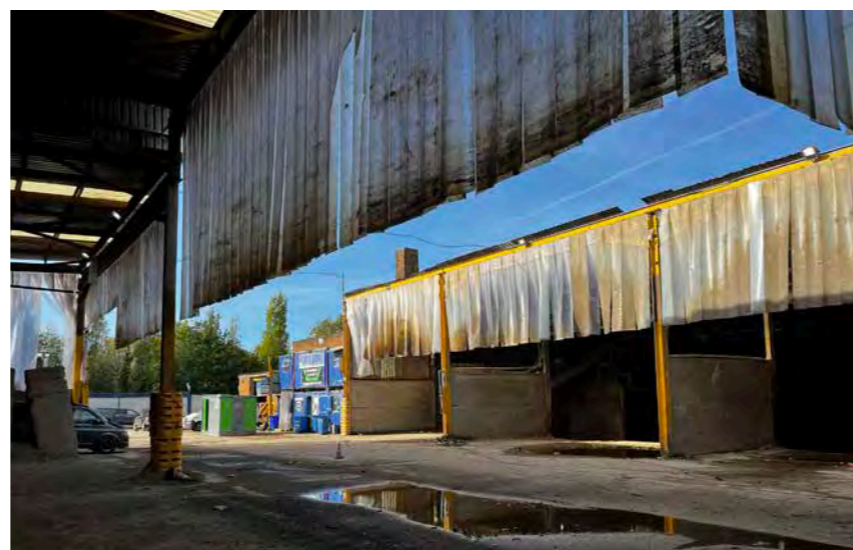
External view of previous waste handling facility
