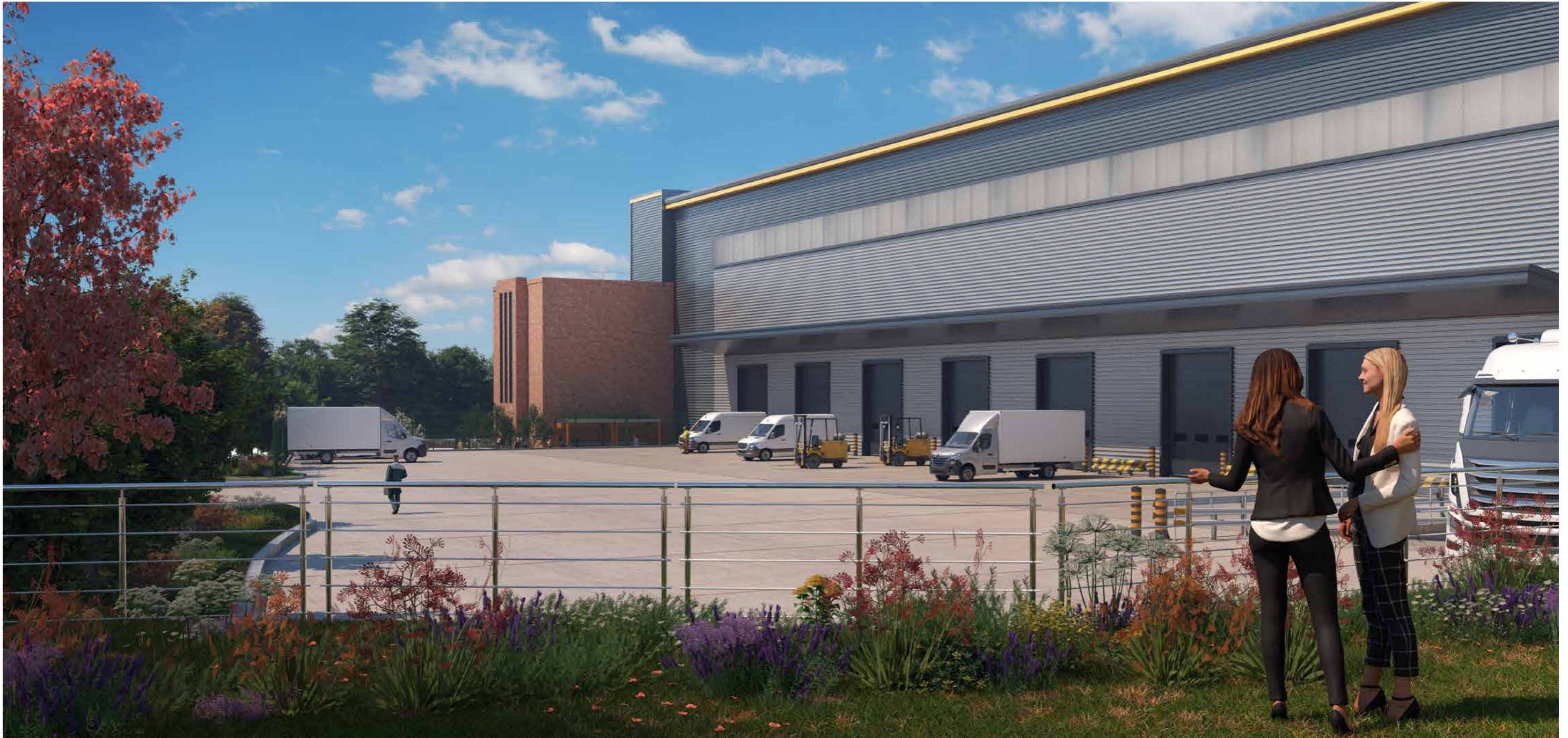
CGI View from southern end of the service yard
