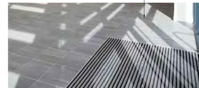
600 x 600mm ceramic floor tiles Grecale - Acciaio Refin Colour Fango with recessed matwell
