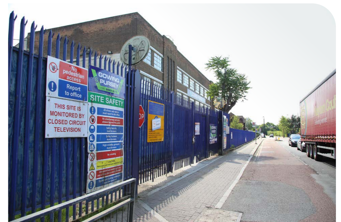
View looking west along Twyford Abbey Road
