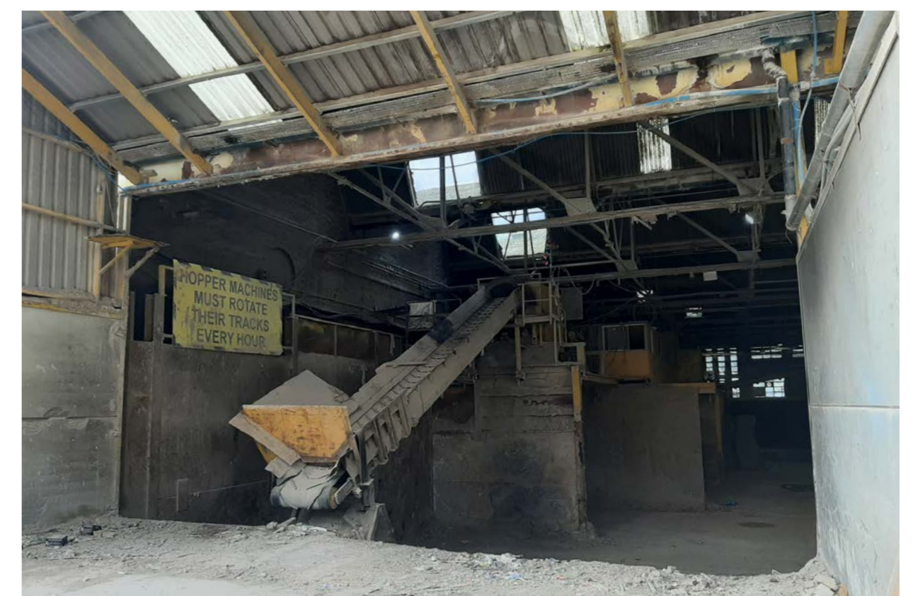
Internal view of existing site
